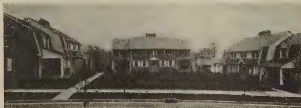
FIG. 13—BUCKMAN VILLAGE, CHESTER, PA.— GROUP OF APARTMENTS G. EDWIN BRUMBAUGH, SIMON & BASSETT, ARCHITECTS
